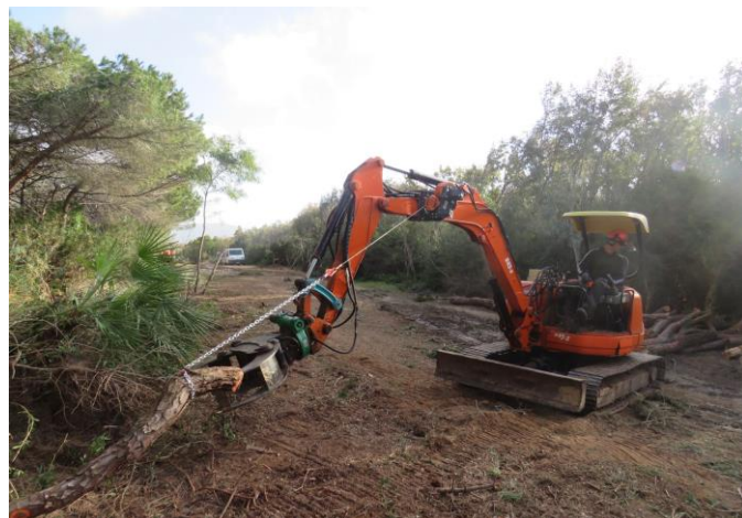
Innovative: motor-manual and excavator+winch
