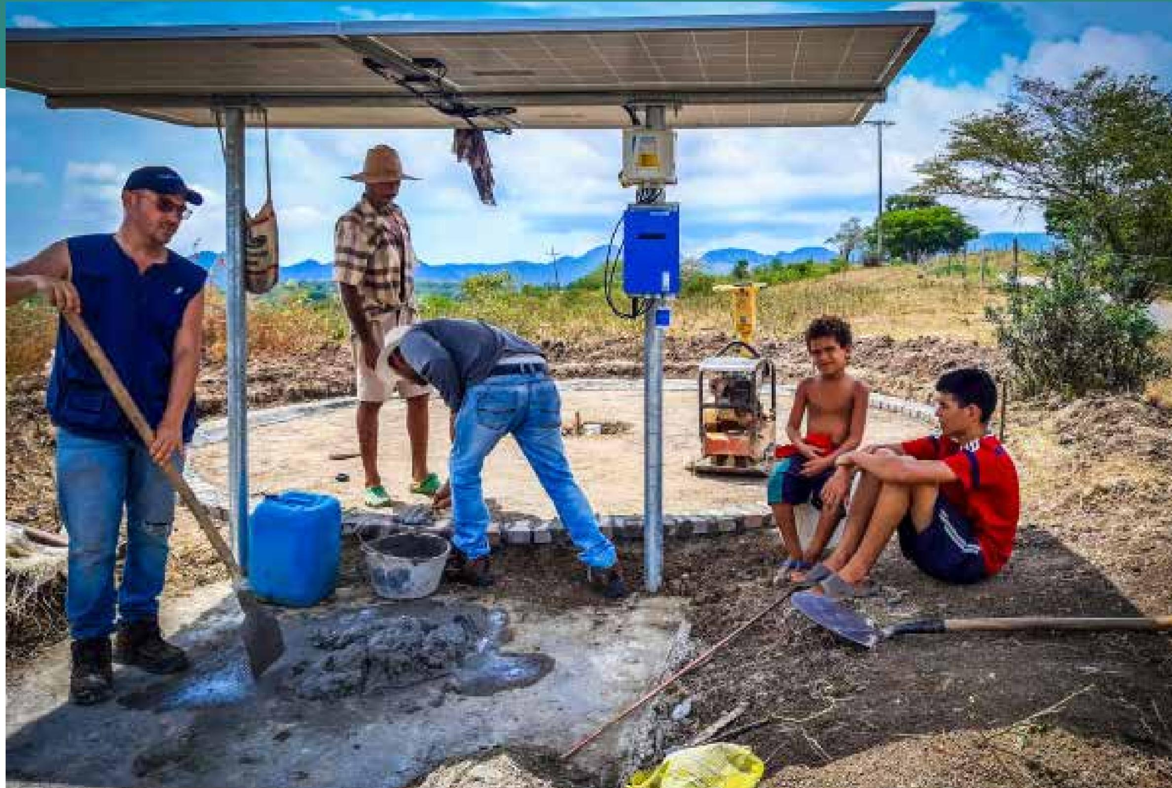
The versatile and space-efficient solar panels serve various purposes. In this case, they provide energy to an electric pump that supplies water from the reservoir.
