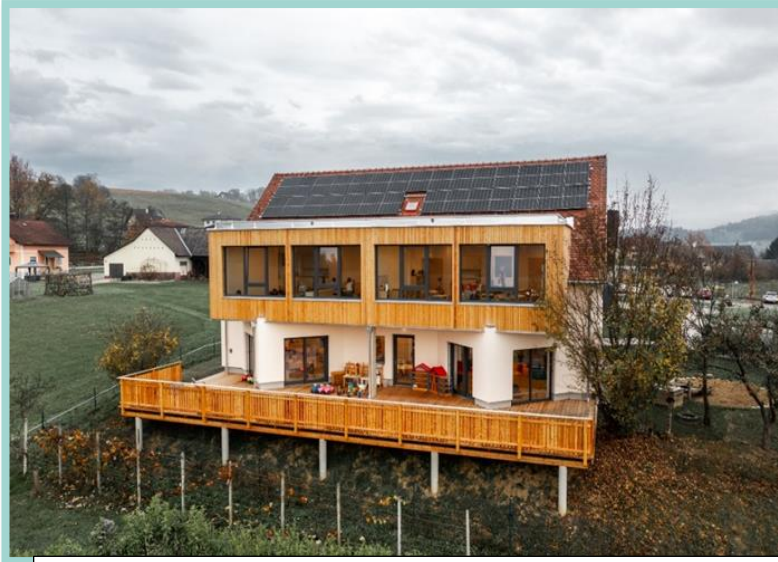
Kindergarten Empersdorf, Austria. Natural materials and architecture with built-in sun protection. Image credit: Daniel Nagler
